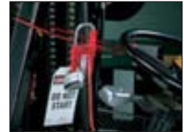
Immobilize large or cumbersome devices, such as forklifts
